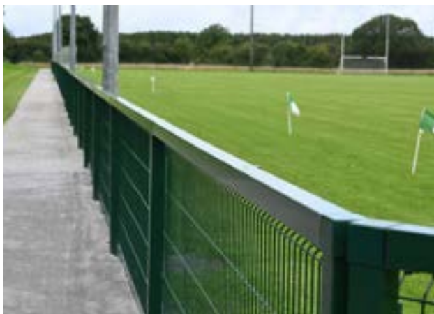
Ballyfore GAA - completed fence.
